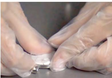
**1** Place and press the clay onto the relevant area. Be careful not to trap air between Ceralun and the base material.
